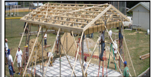
The Kiwanis/NRVHBA Baseball Shelter Build at the Kiwanis Field, Christiansburg, Virginia.
